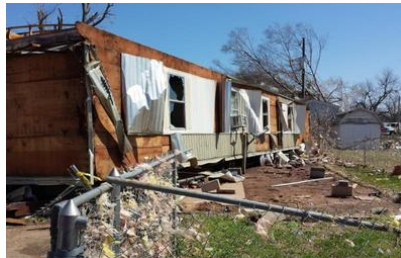
Storm Damage from March 2015 Tornado in Sand Springs
