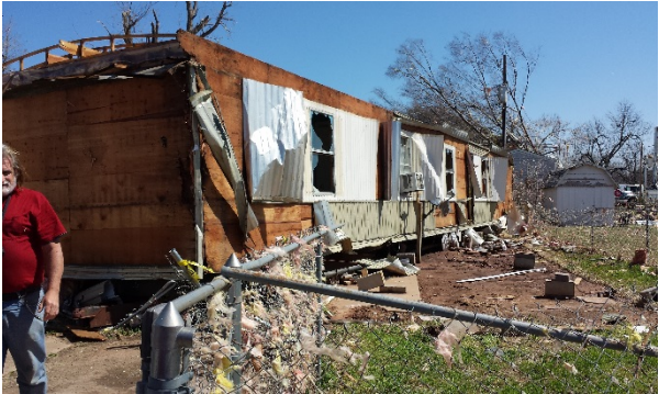
Storm Damage from March 2015 Tornado in Sand Springs, Oklahoma
